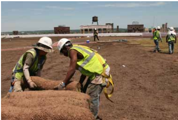
Workers installing sections of the Target Center green roof.
