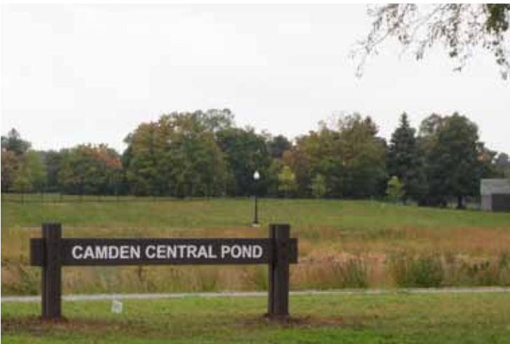
This pond controls flooding and protects Mississippi River water quality by removing significant amounts of sediment and phosphorus from stormwater runoff.
